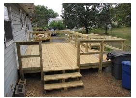
2" x 4" treads on an existing deck and removing the handrails still in-place, completely razing the back 9' of the existing deck, as well as removing an existing ramp to the deck as it was too steep. We then installed additional posts around the new deck footprint and installed new 2" x 6" treads on the shortened 9.5' x 15' deck. The new ramp coming off
