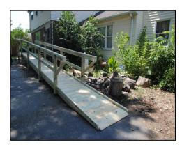
Hunt's project, located in Rosedale, south of the Beltway, included an approximate  $8' \times 6'$  landing over an existing porch and then a 28+' ramp left to the driveway. Typically, a ramp this size would be done in 1 % days. However, due to the forecast of high temperatures with high humidity, the threat of afternoon thunderstorms, the wearing
